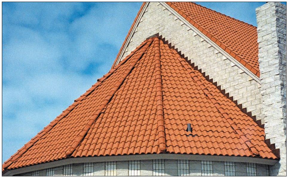
Portions of this intricate roof are both radiused and hipped.
